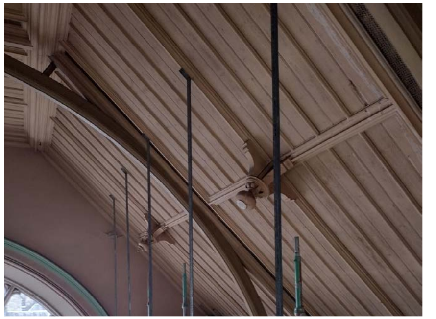
Decorative timber ceiling should not be removed, insulation to be installed from above
