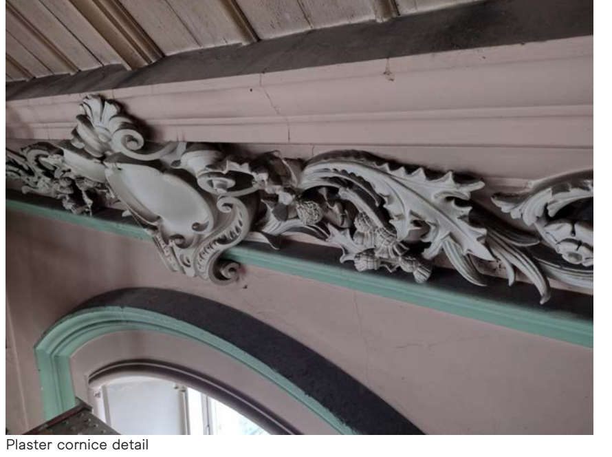
Plaster cornice detail
